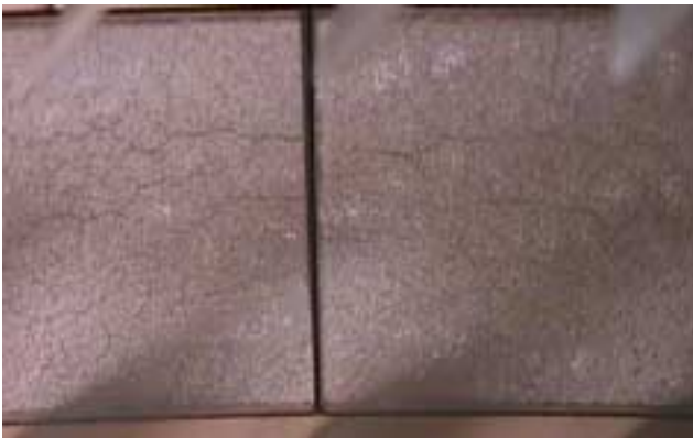
Fig 4 – Cracking of topcoat surface
