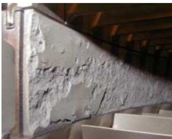
Fig 2 – Missing topcoat not exposing basecoat
