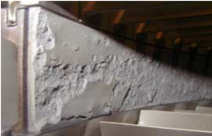
Fig 2 – Missing topcoat not exposing basecoat
