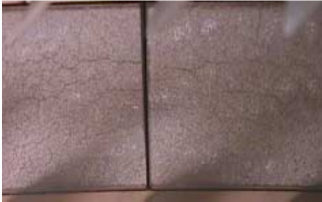
Fig 4 – Cracking of topcoat surface
