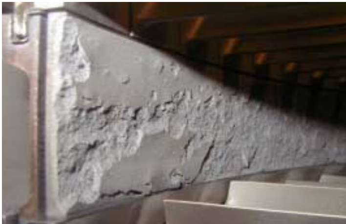
Fig 2 – Missing topcoat not exposing basecoat
