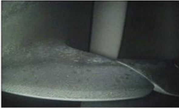
CLAPPERS WITH GOOD ALIGNMENT NO OBVIOUS WEAR
